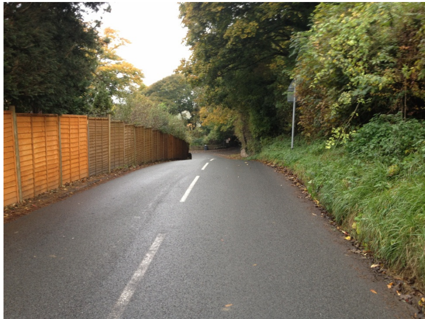
Main Street looking south at narrowing
