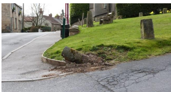
Damage at the Trip Lane triangle
