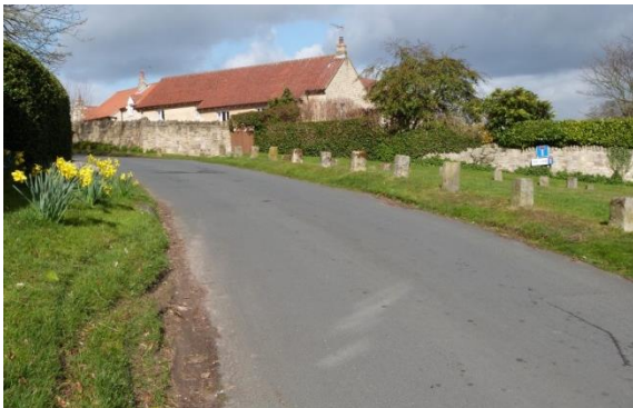
Vehicle damage to grass verges
