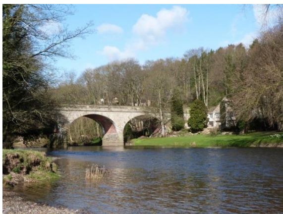
River Wharfe with Bridge
